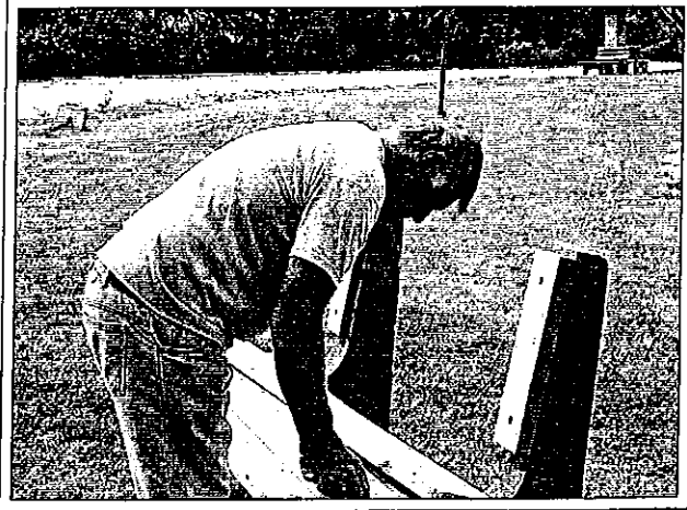
Bench Construction — Jurgen Hendel
