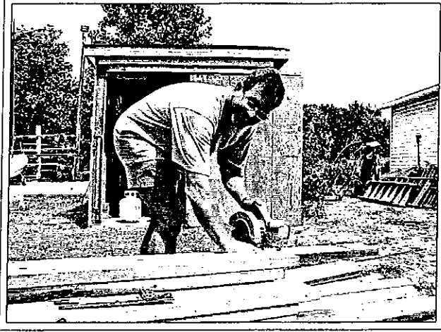
Bench Construction — Steve Kepran
